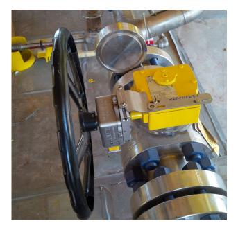
can then be used to open the vessel door safely and load the pig.
