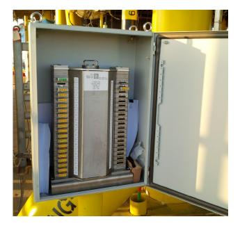
door. To guarantee that procedures are followed, an extra control unit is used in addition to standard valve interlocks. This unit guarantees correct purging procedures, without shortcuts. For example, when a vessel needs to be purged 7 times, the mechanical control unit is programmed to force operators to purge 7 times before opening the vessel. These steps cannot be skipped This will keep the integrity of the plant and the safety of the operator a priority.
