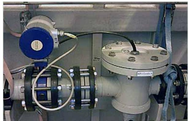
Installed sonic velocity and conductivity sensor
