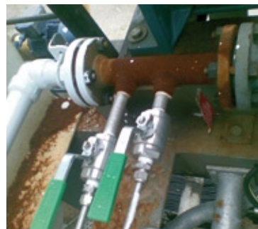
3 - V-Cone in Carbon Steel DN 25 flangiato in curva
